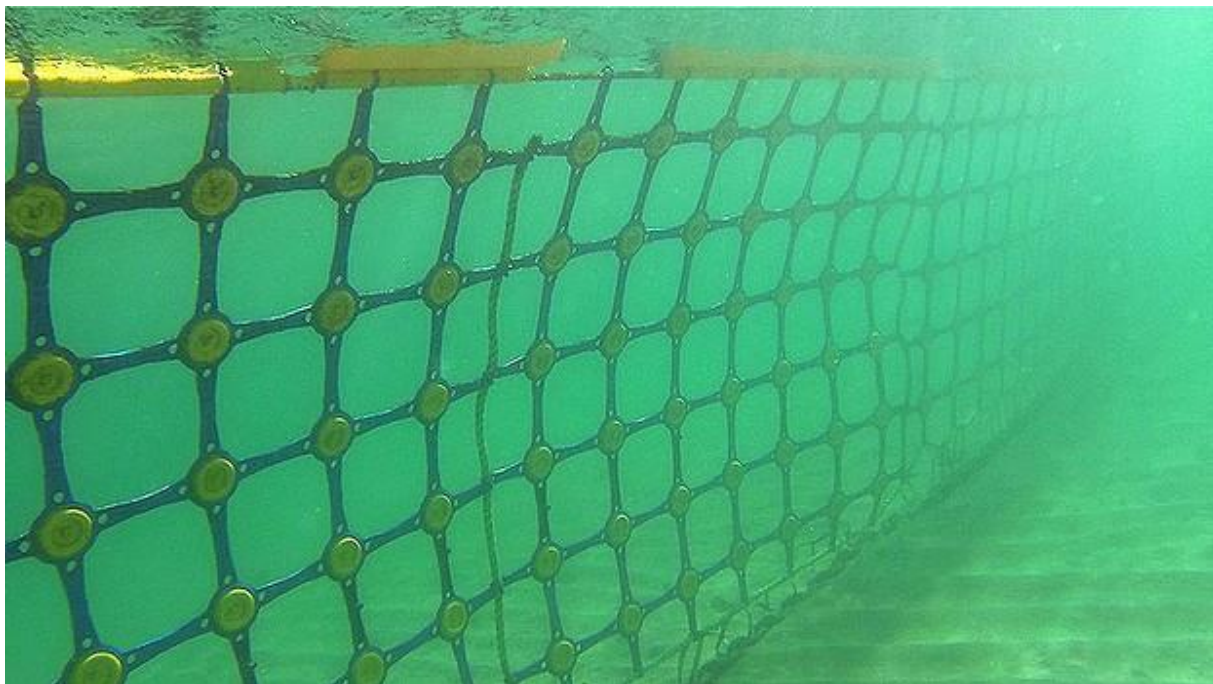
Figure A1-4 Section of interlocking Eco Shark Barrier installed at Coogee beach (WA Today, 2014)
