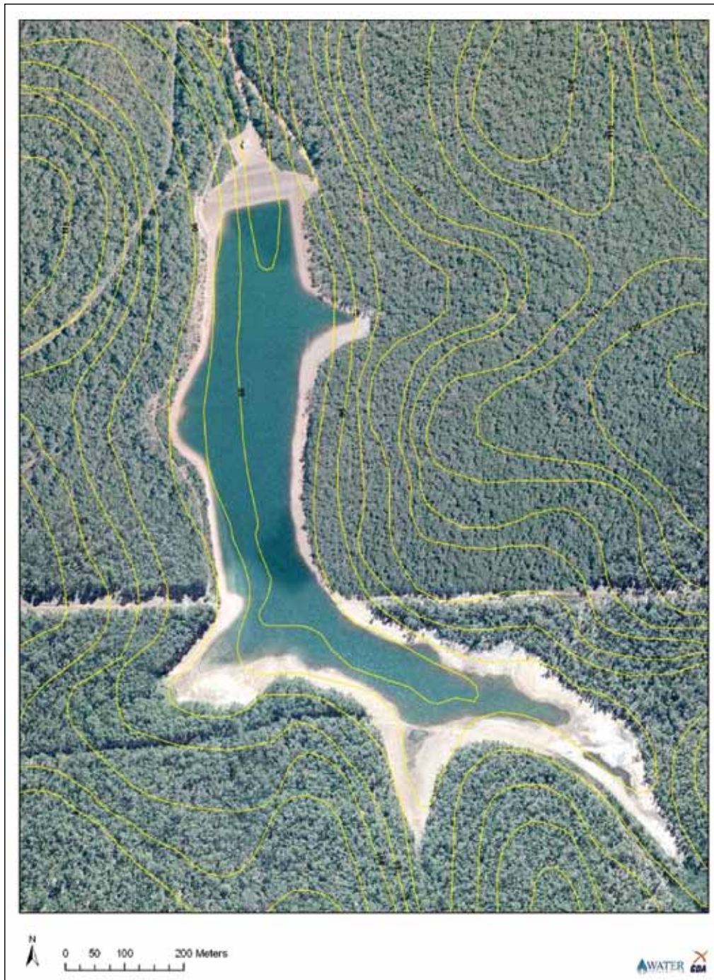
Figure 1. Ten Mile Brook Dam (Figure courtesy of Water Corporation).
