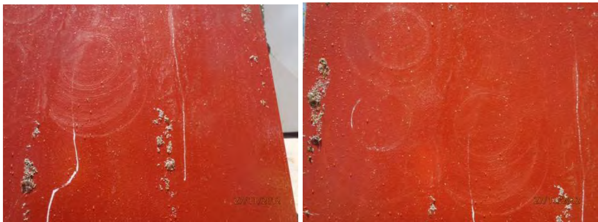
Figure 5.4 Scuffing of the coating surface caused by the blades touching the surface.
