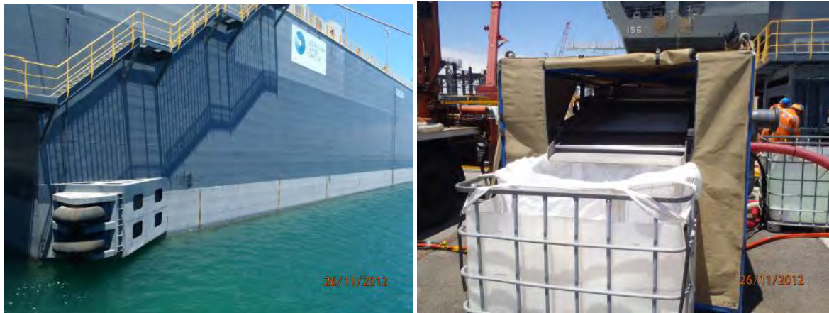
Figure 4.1 Dry-dock Yargan (left), and first stage filtration unit (right).
