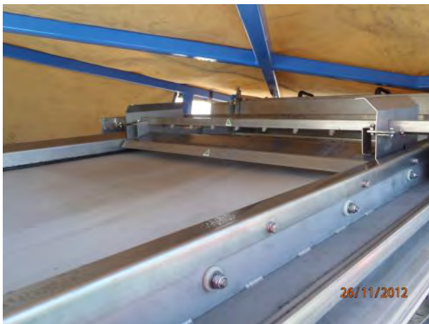
Figure 2.6 First stage filtration: filter screen
