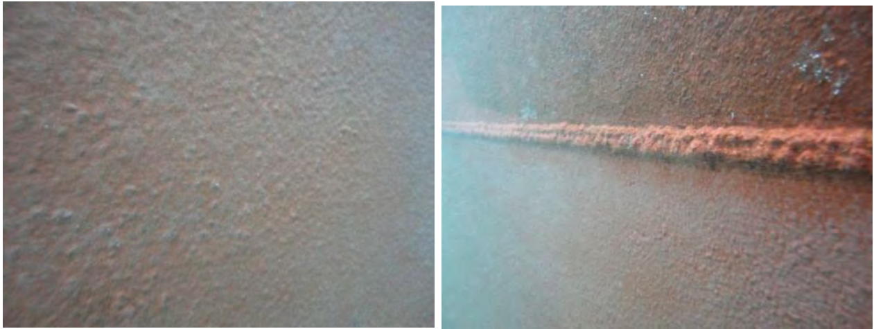
Figure 6.4 Hull surface after cleaning with the Envirocart fitted with bladed discs.
