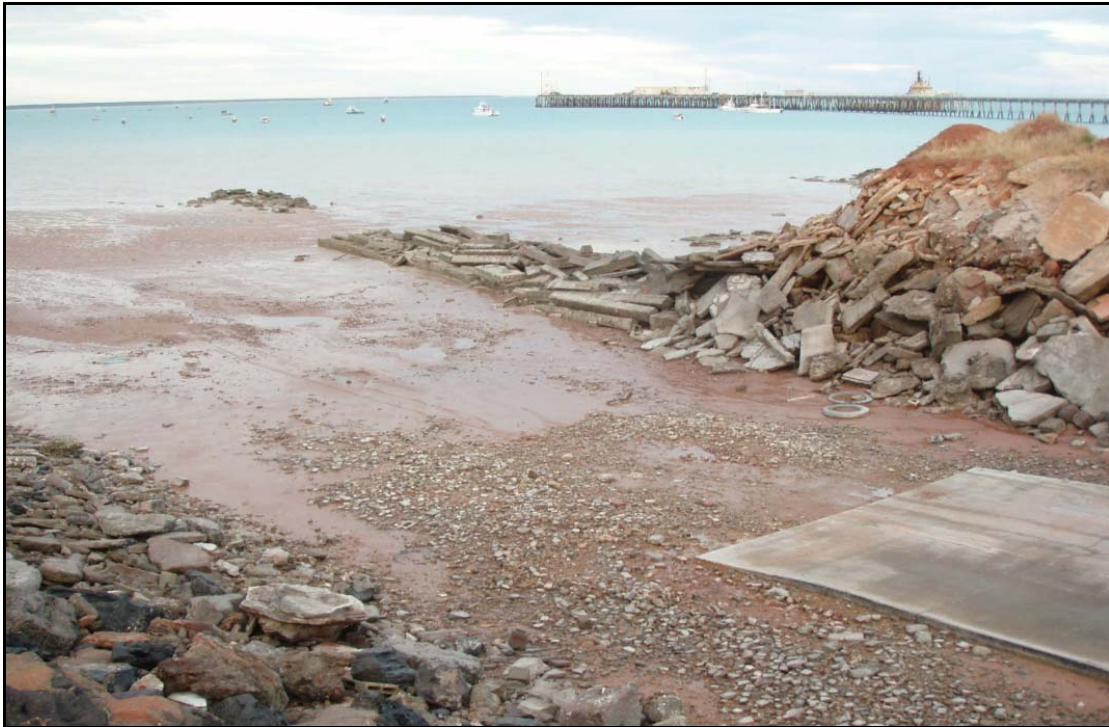
Figure 6. Boat ramp associated with Broome hard stand area
