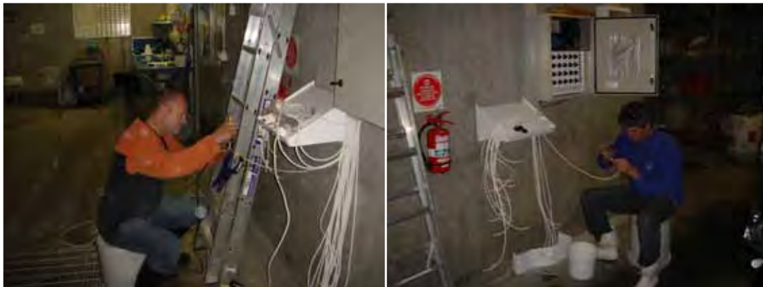
Figures 1-2. DoFWA staff installing the system.
