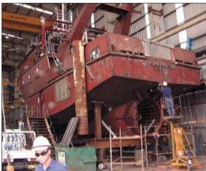
The RV Naturaliste under construction. The RV Naturaliste will replace the RV Flinders. RV Naturaliste was built during the later part of 2000/2001.
