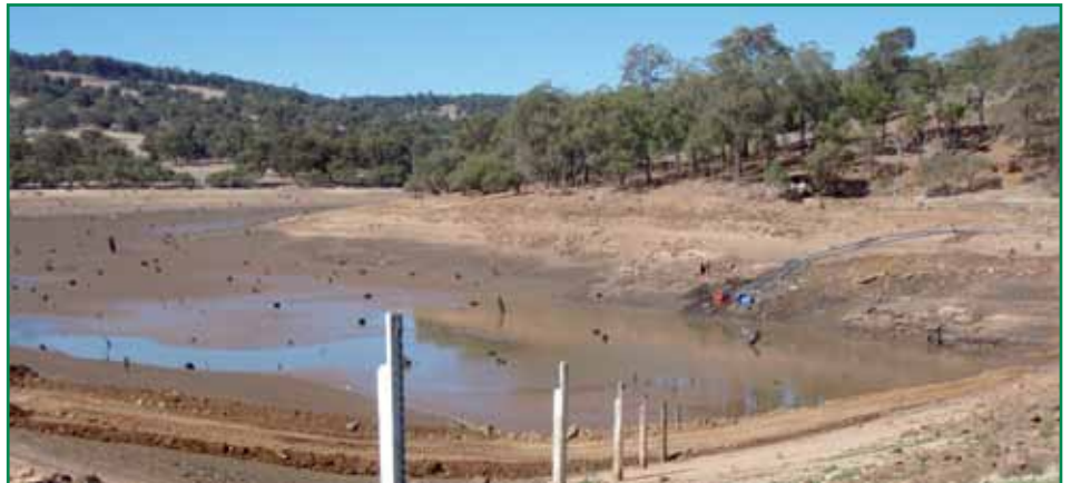
A dry Drakesbrook Weir.
