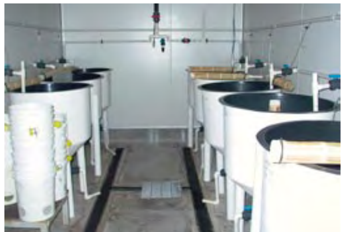
Figure 3. Eight 220L egg incubation tanks adjacent to the broodstock room in the SARDI R&D Hatchery.
