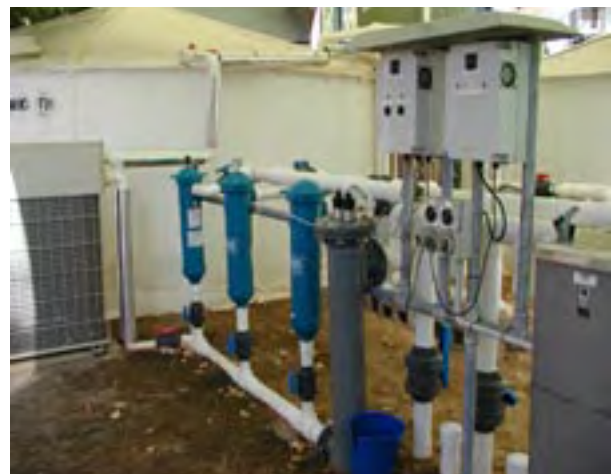
Figure 2. Primary water treatment for "new" incoming water including bag filtration, UV sterilizers, heat exchanger
