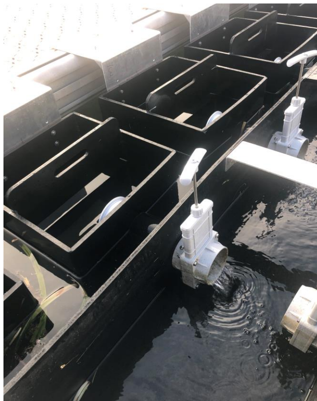
6 Central gutter showing maximum flow through the upwellers.
